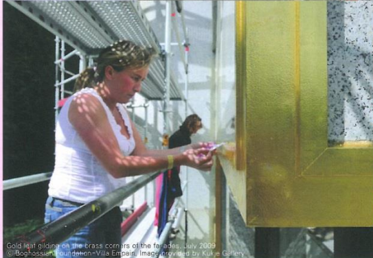
Gold leaf gilding on the brass cornices of the balconies, July, 2009 © Boghossian Foundation-Villa Empain, Image provided by Kukje Gallery
